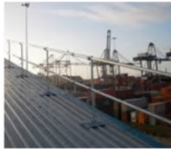
Edge Protection on Pitched Roof
